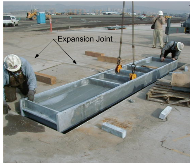
Beam Installation
