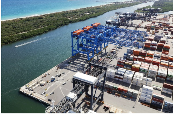
New cranes in blue operating with existing cranes
