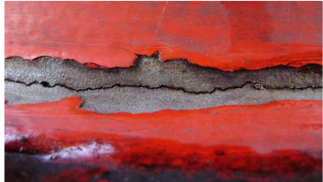
2. End pipe stub column at bolted flange plate
